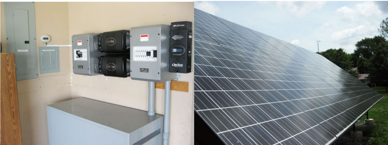
3.3KW Grid solar system (Residential)
